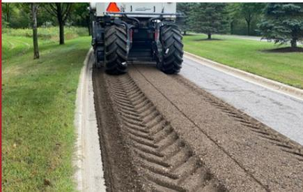
Grind existing pavement and gravel base into a new uniform base material. Grade and compact, then pave new layer of asphalt.
