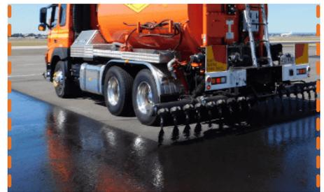
Apply a new coating (or seal) to pavement to provide protection against sun, water, oils, salt and other damaging elements.
