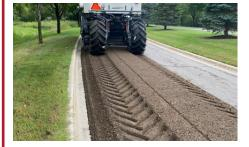
Grind existing pavement and gravel base into a new uniform base material. Grade and compact, then pave new layer of asphalt.
